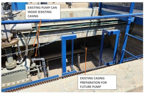
Existing casing for installation of the new pump (NPSHa given at the marked level):
